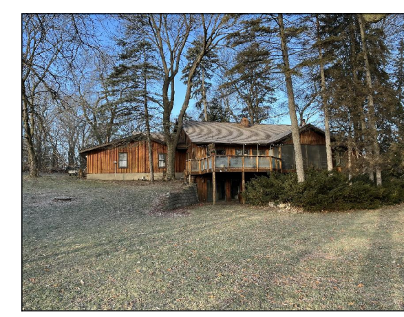
REAR OF 1639 14TH AVENUE N.W. CITY OF NEW BRIGHTON, RAMSEY COUNTY, MN
