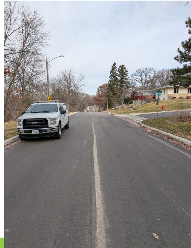
20 th Avenue SW
