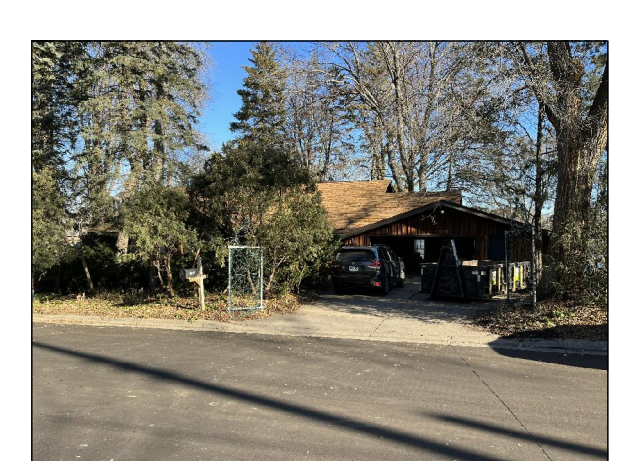
FRONT OF 1639 14TH AVENUE N.W. CITY OF NEW BRIGHTON, RAMSEY COUNTY, MN
