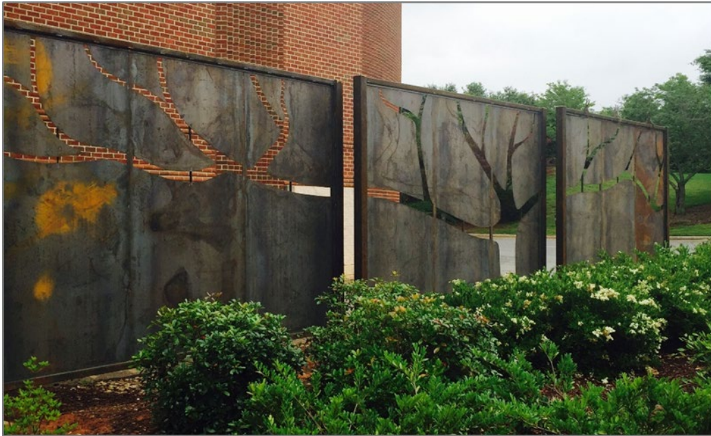
Figure 3-6: Screening walls with landscaped buffers are required around all otherwise visible loading docks, utility structures, and service areas. Creative integration of public art as part of the screening (as shown here) is encouraged.
