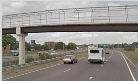
Pedestrian Bridge over Hwy 100
